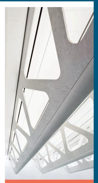
With no storage space and no time to build on site, ROCKFON ceiling panels were cut in custom sizes and mounted to the modular trusses in an off-site location. These pre-fabricated units were then were trucked to the site and installed at night to minimize disruption. The recreation center remained open for business throughout construction.
