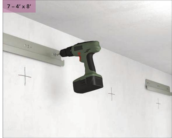
Drill the holes and install the wall bracket.
