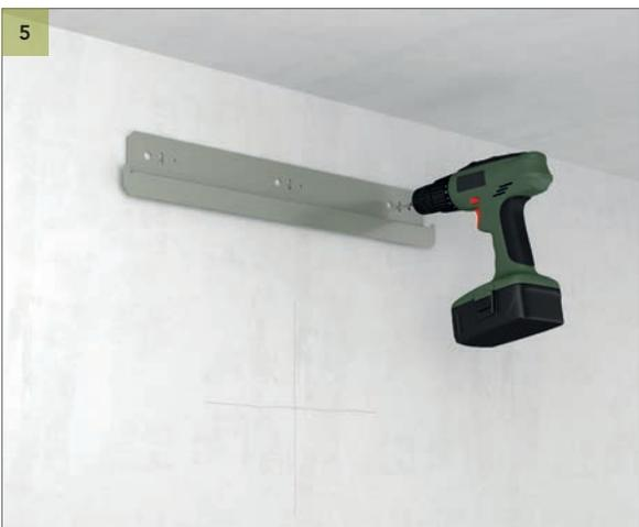
5 Drill the holes and install the wall bracket.
