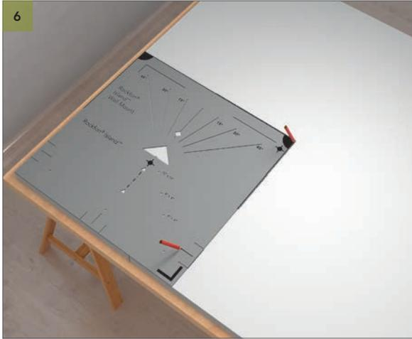
Position the marking tool in the lower left corner on the back side of the Rockfon® Island™. Mark with a pencil the center lines, using the upper right corner of the marking tool, and the position of the spacer. See 7.
