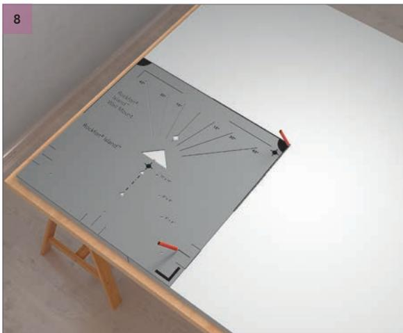
Position the marking tool in the lower left corner on the back side of the Rockfon® Island™. Mark with a pencil the center lines, using the upper right corner of the marking tool, and the position of the spacer. See 9.
