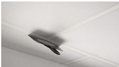
Load the thinned edge with Powder Filler.
