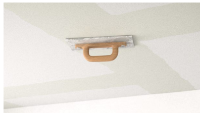
Sand joint down manually.
