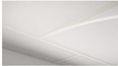
While the Filler is still wet, position the tape on the joints.
