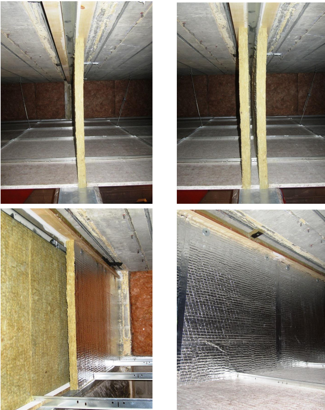
Fig. 2 - Lightweight, stone wool, plenum barriers installed above the central demising wall of the laboratory's chamber during some tests. Top-left: Single-layer. Top-right: Double-layer with a 42 mm (1-5/8 inches) airspace in between. Bottom-left: Double-layer with seams staggered and small cuts at the bottom so the panels slide down over the grid bulb. Bottom-right: Intallation complete with tops screwed, seams taped and ceiling panels installed.
