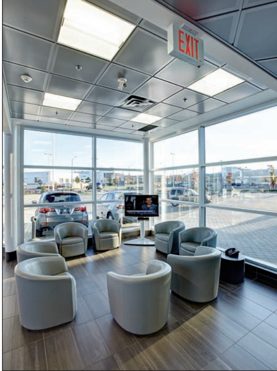
Metal ceiling panels may be perforated in one of many different perforation pattern options for increased acoustical performance and visual variety. For this Acura dealership (Maple, Ont.) lay-in metal ceiling panels also integrate with industry-standard lighting and air-diffusers.
