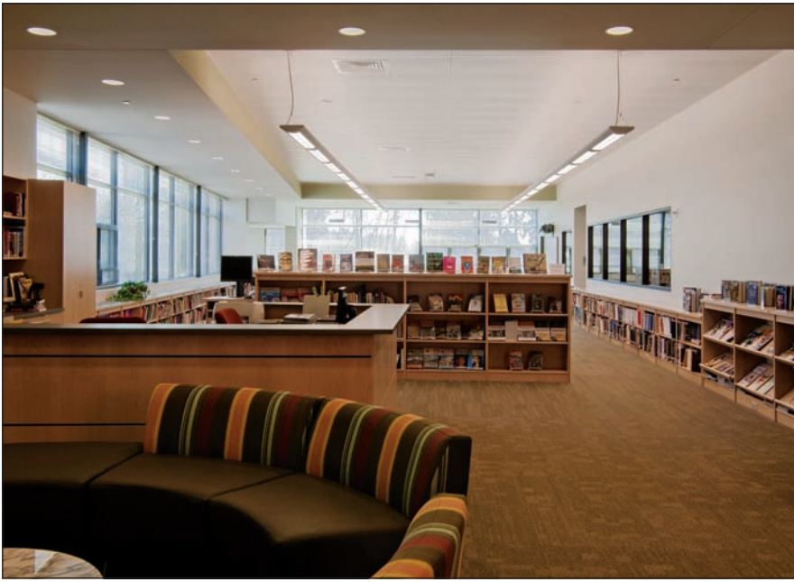
Metal ceiling panels contribute to creating quiet, comfortable learning environments and low maintenance. These hooked-in planks were specified with acoustical performance enhancements and painted white for a light-softening effect. They are easily removed for accessibility to mechanical and electrical services in the plenum.
