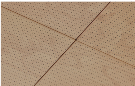
The lobby of John Michael Flaherty Building in Ottawa, Canada. Plank hook-on metal panels have an acoustic backer and closely spaced perforations to optimize acoustics, while mimicking the look of natural wood with painted finishes. Photos courtesy of ROCKFON/Bochsler Creative Photography.
