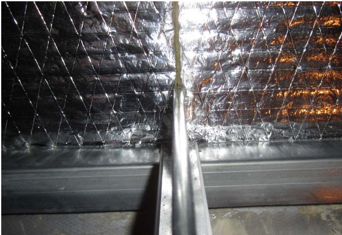
**Figure 9: A close-up of a stone wool plenum barrier installed over an interior partition. The pliability of the material lets it conform around elements, such as the ceiling suspension system's main runner, and along uneven adjacent surfaces, such as the top track of the partition, without leaving gaps and openings. Typically, no caulking is required.**
