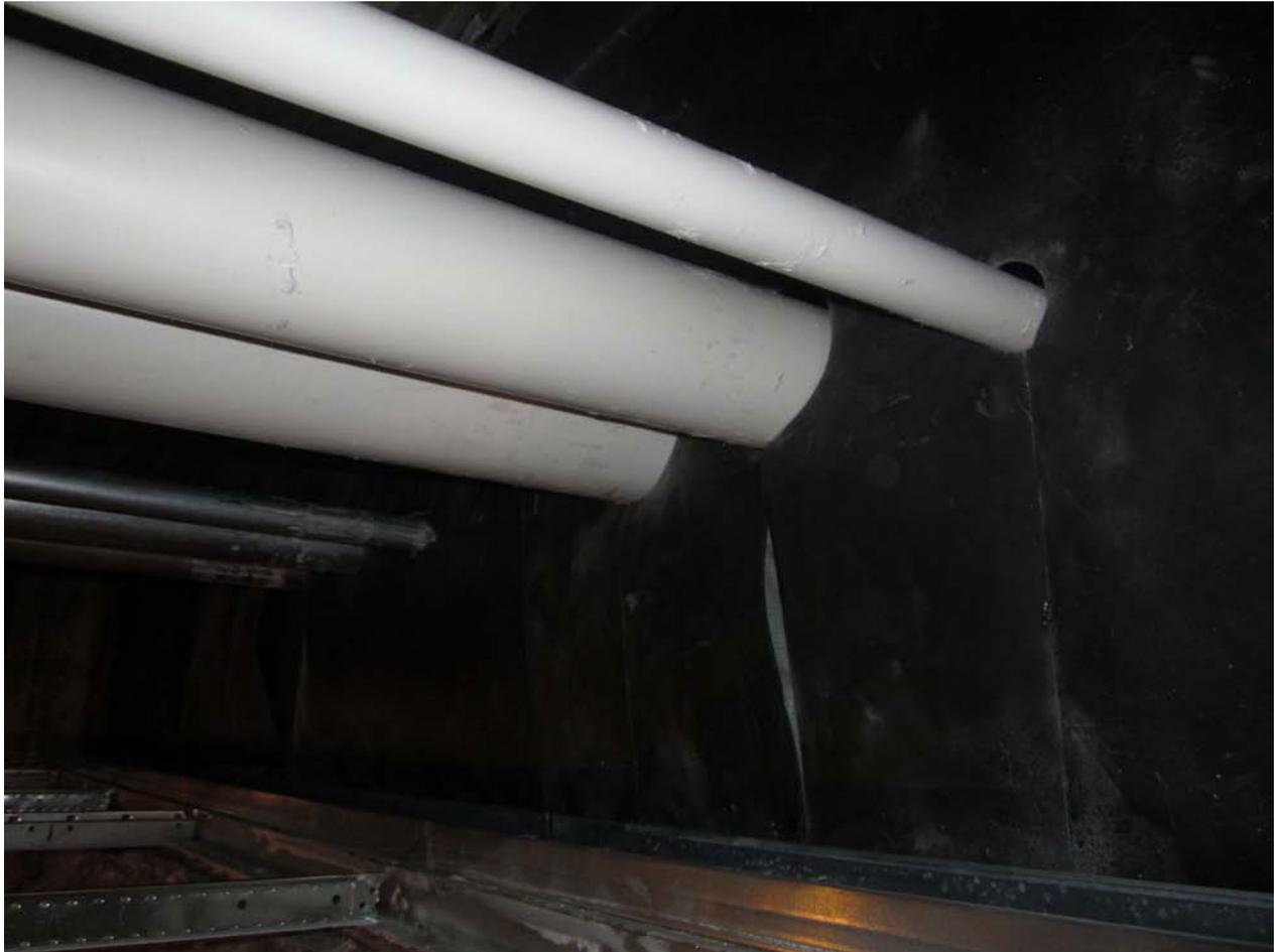
**Figure 6: A MLV plenum barrier is installed above an interior partition. The memory of the material causes it to curl, pulling the material away from the taped seams and resulting in openings in the barrier. Because the material is thin and smooth, caulking gaps around penetrating elements is not possible.**
