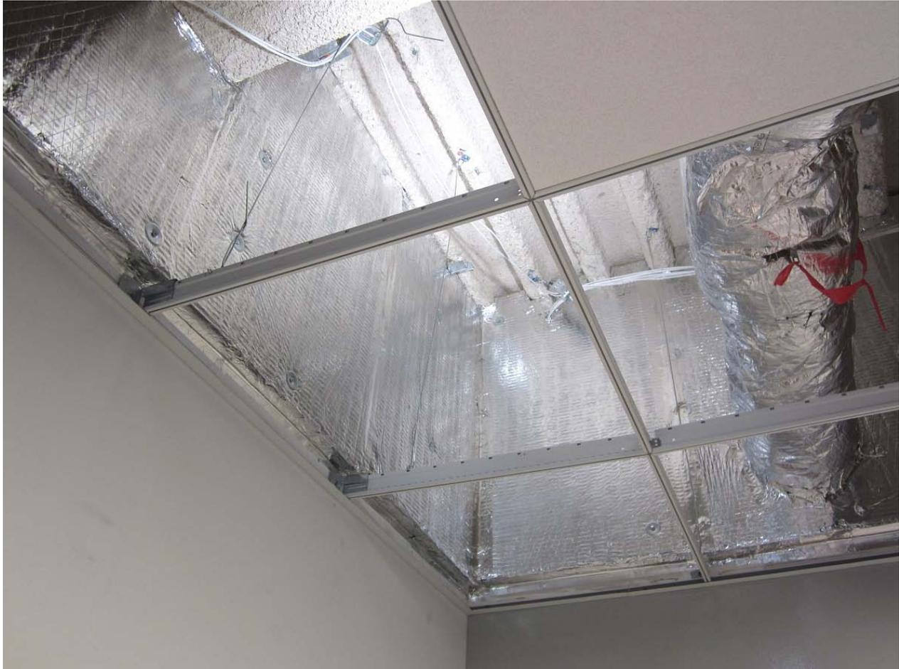
**Figure 2: A private office inside a commercial interior fitout. View from below the acoustical ceiling with some ceiling panels removed to show the plenum barriers above partitions that terminate at ceiling height. The plenum barriers block noise that would otherwise transmit through the ceiling and over the top of partition.**
