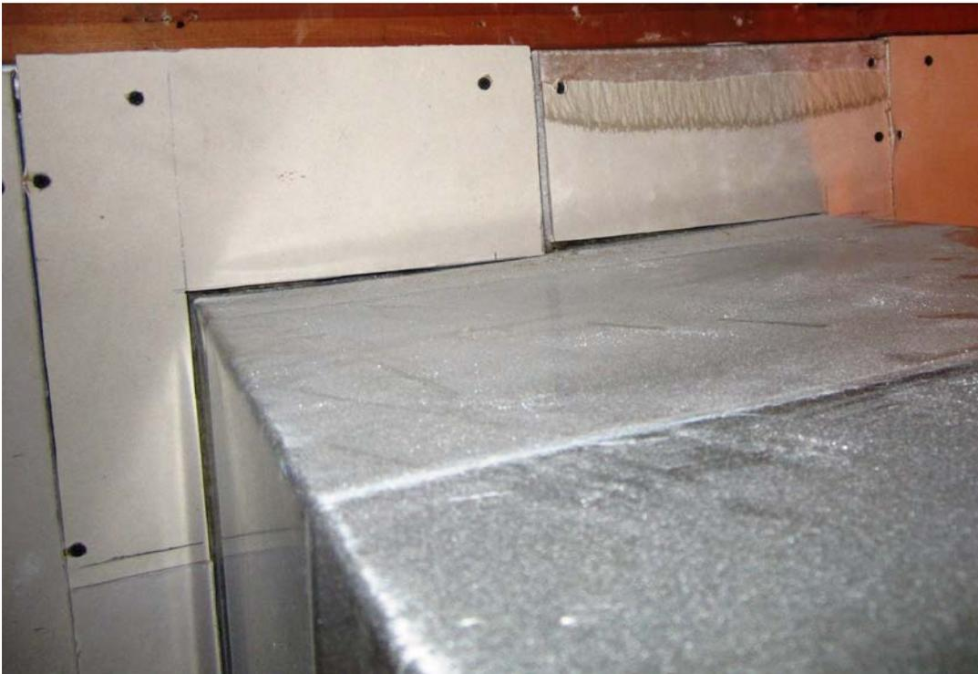
**Figure 7: Part of a gypsum board plenum barrier is installed around a supply air duct. The rigidity of the material combined with the imprecise score-and-snap method of cutting the material result in many small gaps and openings.**
