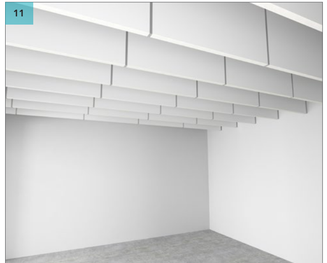
Fissare i restanti Rockfon Industrial Baffles.
