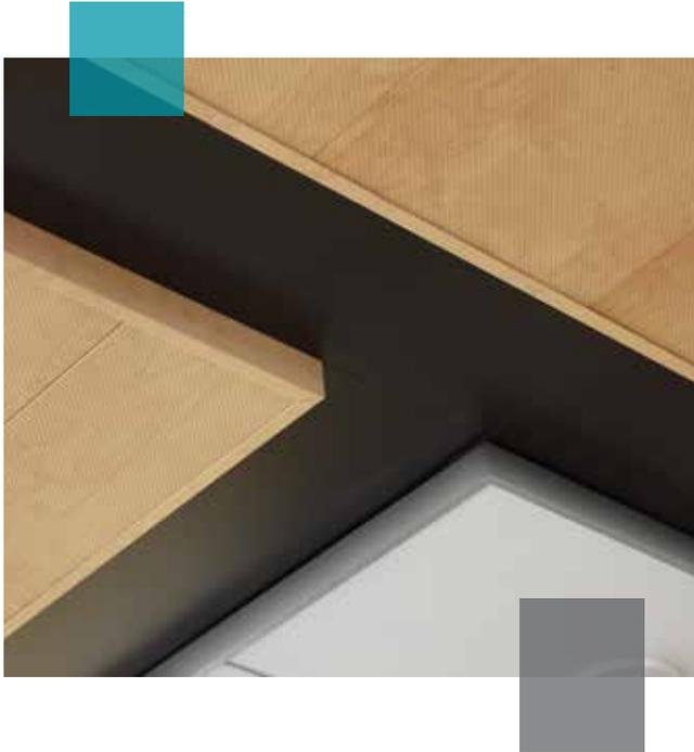
Accommodating the lights and air diffusers, the custom-sized Planostile planks were finished in both black and in Satin Silver. The Satin Silver was matched with Rockfon Infinity perimeter trim for a clean, smooth edge. Beyond the numerous sizes of factory-cut panels, the large columns in the main lobby also proved challenging.
