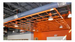
The Rockfon® Cubegrid® Open Plenum 15/16" Ceiling System uses standard grid suspension that has been specifically manufactured with all extra holes and slots removed, allowing for a high-quality architectural finish on all sides. This easy-to-install, cost-effective, open ceiling system can be used to mask the plenum or highlight a specific space. Integral cross tee couplings, combined with no visible hanger slots and holes, makes Cubegrid the cleanest open cell ceiling suspension available.
